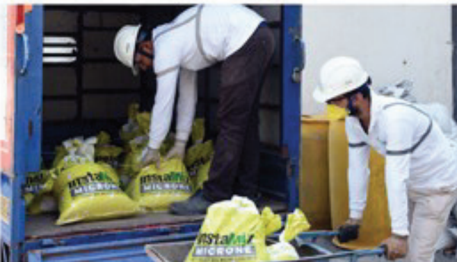
Unload the Microne bags from vehicle and stack near pouring area
