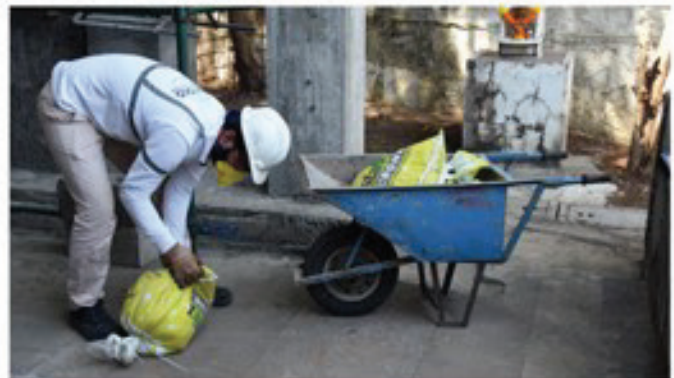
Shake well the Microne bags before pouring
