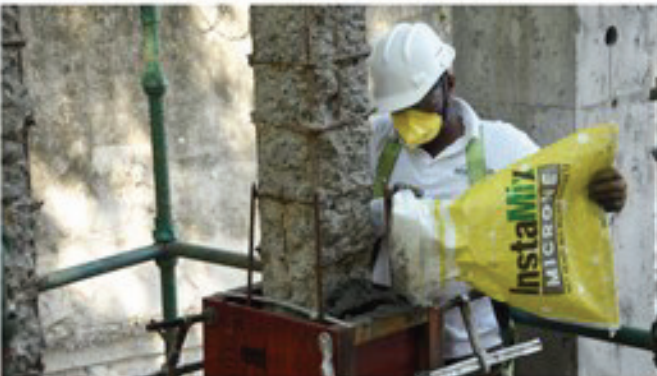
Open the bag and directly pour the Microne in jacketing
